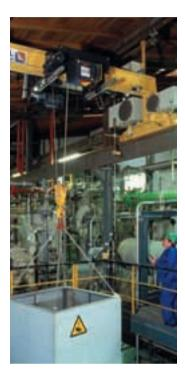
designed for working in hazardous areas and meets the ATEX requirements for Zone 1 or Zone 2 or Zones 21 or 22. The basis is the field-proven SH wire rope hoist programme which ranks among the most outstanding and extensive product ranges available internationally. All components come from a single supplier and our own manufacture.
